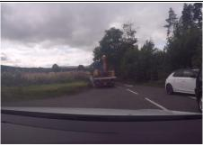
The junction between the A862 and A833 is too small currently to allow the AIL to pass. Significant road widening is required which extents out with the highway boundary. This requires the removal of the small walls which delineate the bell mouth to the A833.
