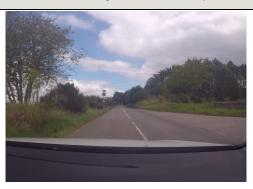
The AIL heads west along the A831 past the existing Beauly sub-station. The carriageway cross section is of a reasonable standard and no modification works are required. The AIL will require the full cross section of the road.
