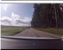
The B9169 has lane widths of approximately 3.3m and total cross section width of 6.6m-6.8m. The AIL will need the full width of the road, therefore, traffic will need to be held in Muir of Ord.
