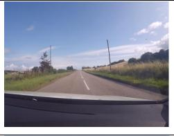
The B9175 is of a good horizontal standard and has a suitable cross section for the AIL. There are numerous overhead services along the route (electricity and openreach). These appear to be at suitable clearance so not to impact the AIL. however, targeted survey will be required to confirm this.
