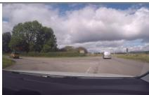
The junction with the A832 to the B9169 shouldn't require any modification. It is proposed the AIL maintains its direction on the A832 heading west and then manoeuvres into the B9169 using the existing informal widening which is already present at the junction. The suitability of this movement should be confirmed with the appointed haulage contractor as it likely needs a change of direction of the tractors pulling and pushing the load.
