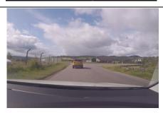
The junction with the B9169 and A862 requires widening into the nearside verge to allow the AIL to pass safely. There may also be interaction with a small wall on the northbound verge of the B9169 which may need to be removed to facilitate the load passing. This will need to be confirmed by the specialist haulage company.
