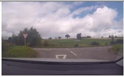
The existing junction on the A831 needs some reasonably substantial widening to facilitate the load passing through. There is existing communications chambers and cabinets which will require re-located to allow the AIL to safely negotiate the junction. The widening to the north of the junction extents outwith the highway boundary into private land which will require consultation and agreement with the landowner.
