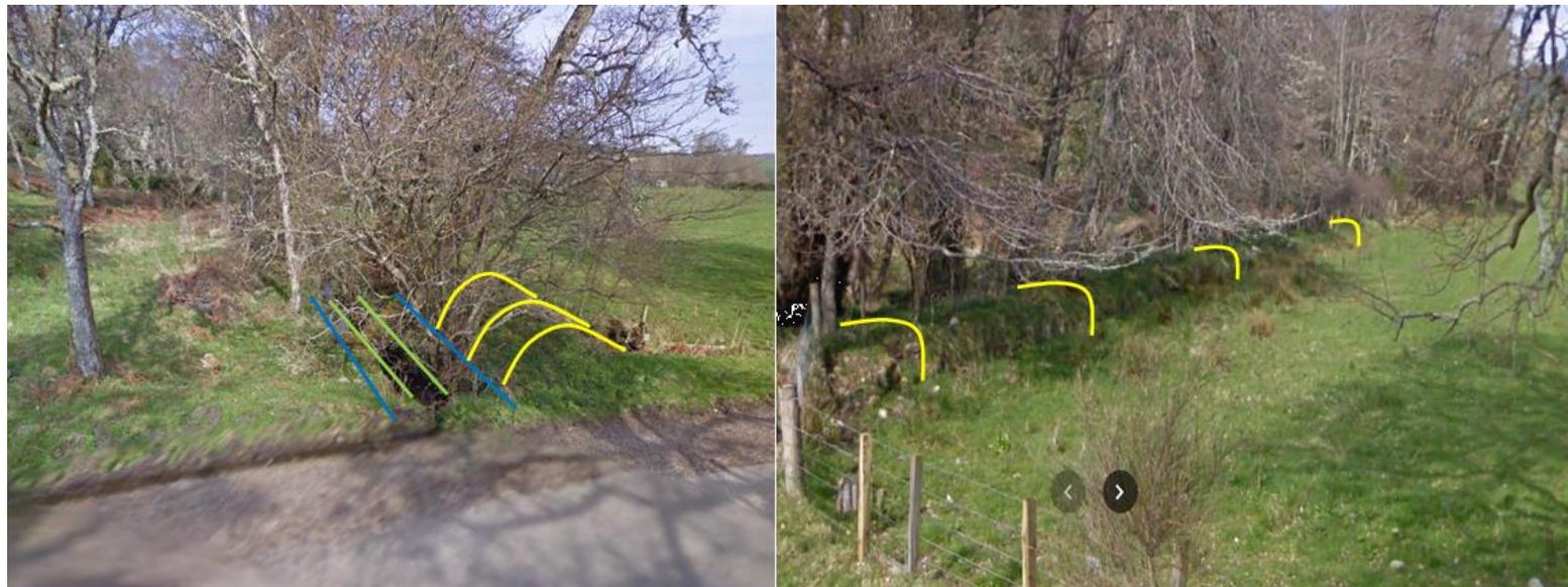
Figure A-1 images used for assumptions about channel and embankment geometry. Blue line = top of bank. Green line = toe of channel. Yellow line = embankment
