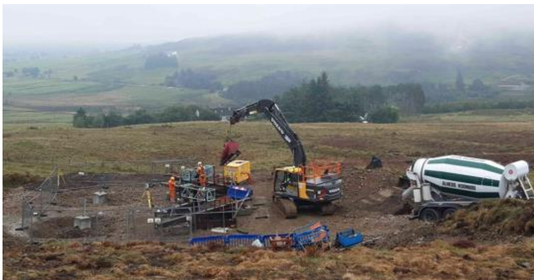
Photo 3.1 Illustrative Image of Tower Foundation Construction
