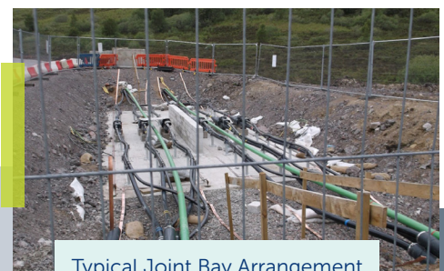
Typical Joint Bay Arrangement
