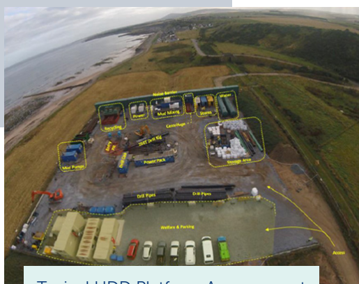
Typical HDD Platform Arrangement
