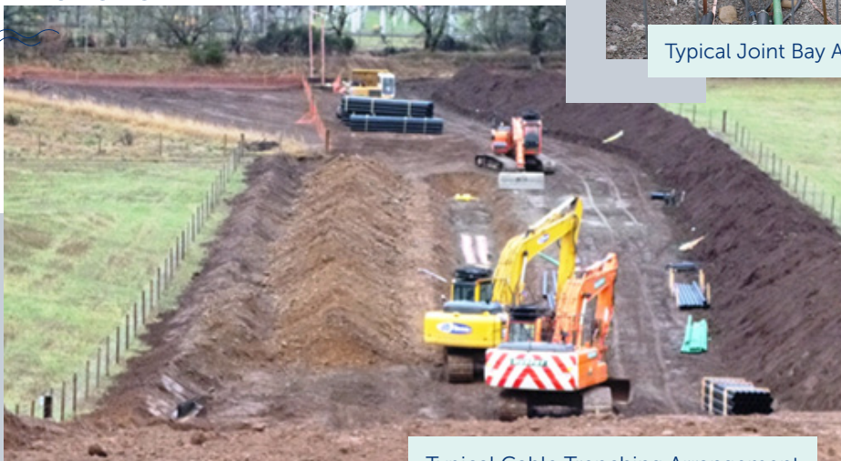
Typical Cable Trenching Arrangement
