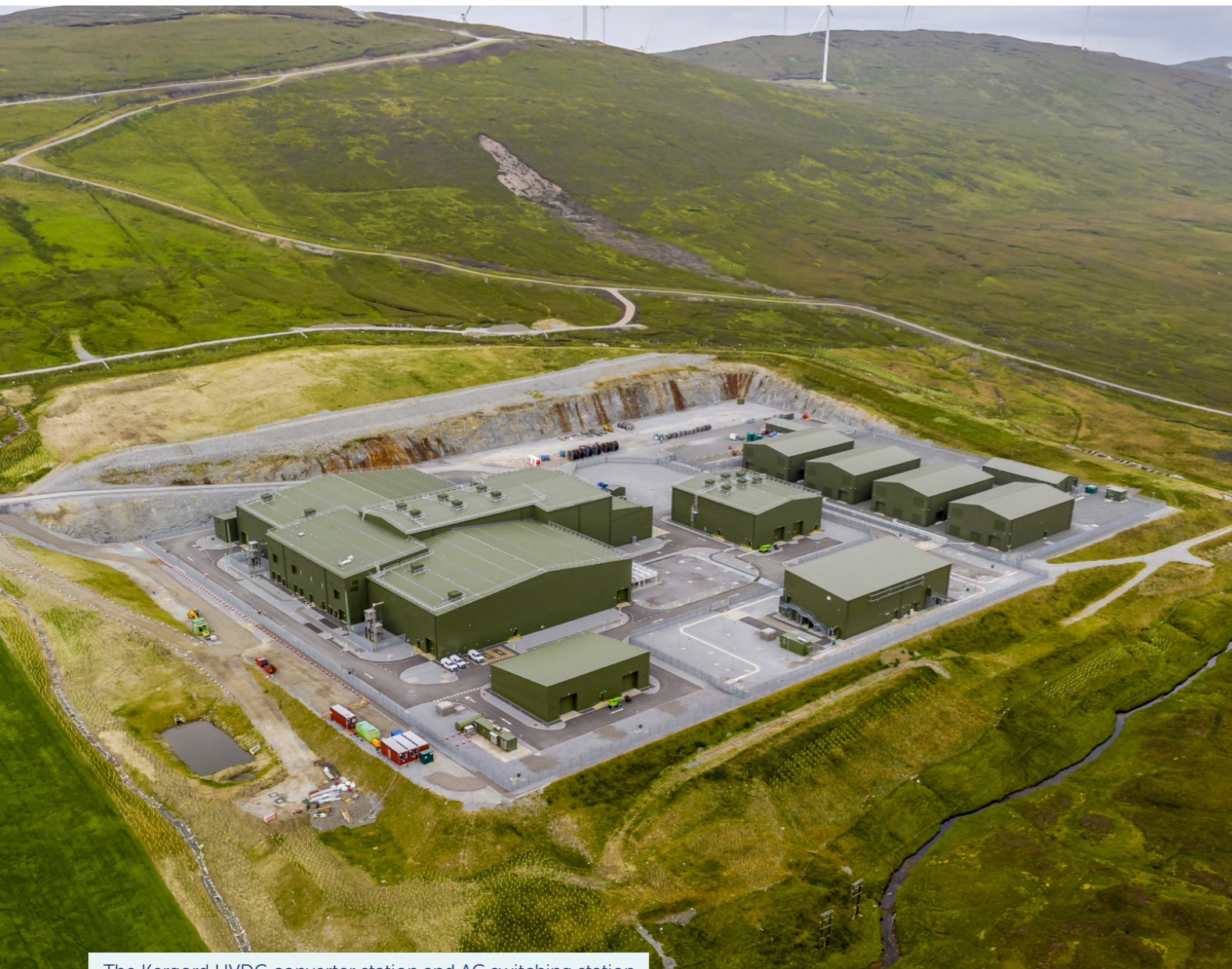
The Kergord HVDC converter station and AC switching station
