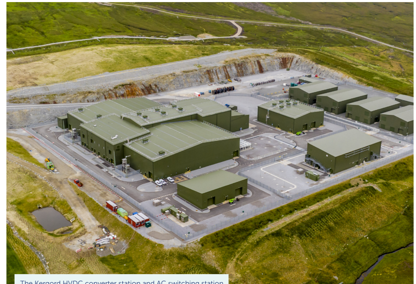
The Kergord HVDC converter station and AC switching station
