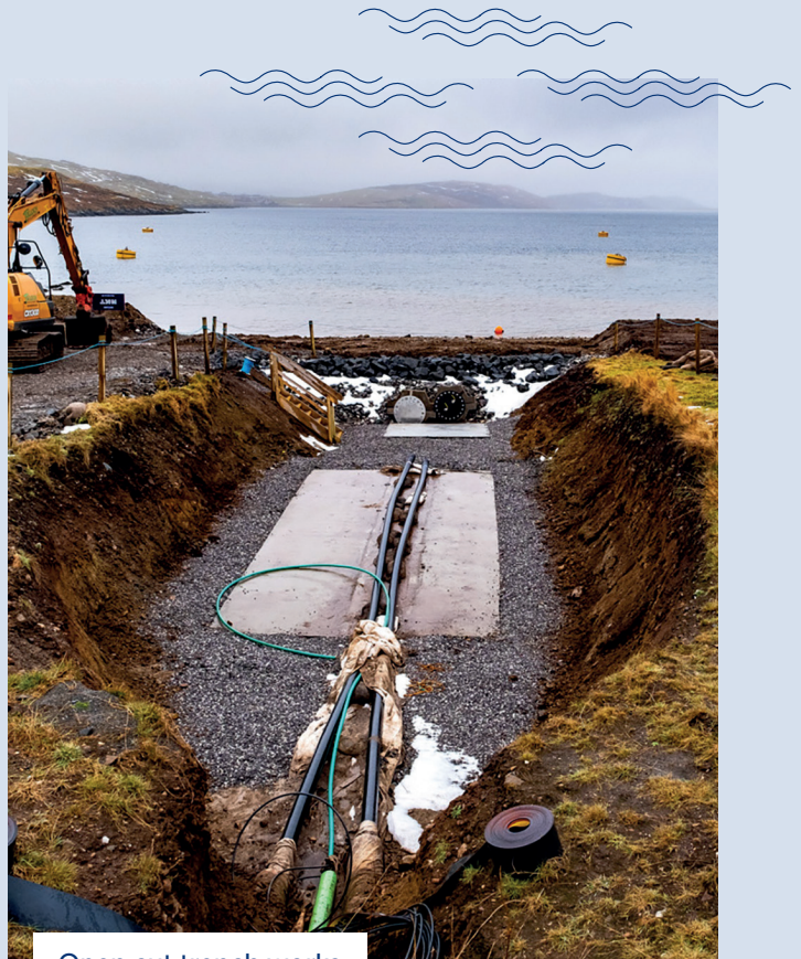
Open cut trench works
