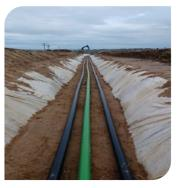
UCG power cables; either ducted or directly buried, in an underground trench nominally
