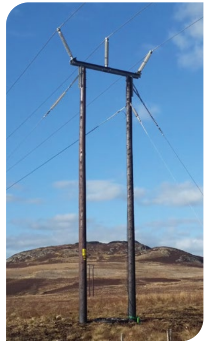
Construction of a 'H' Pole
