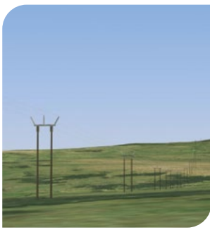
Single Circuit Trident Low Profile OHL. Standard Pole height is between 11-17m and pole spacings are in the range 70-100m.
