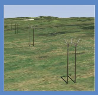
The preferred solution is single circuit trident wood pole with traditional and new technology conductors, although sections of alternative technology, eg underground cable and alternative supports, may be required in some areas to accommodate environmental and technical constraints.
