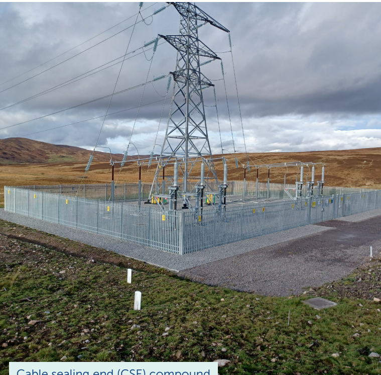
Cable sealing end (CSE) compound
