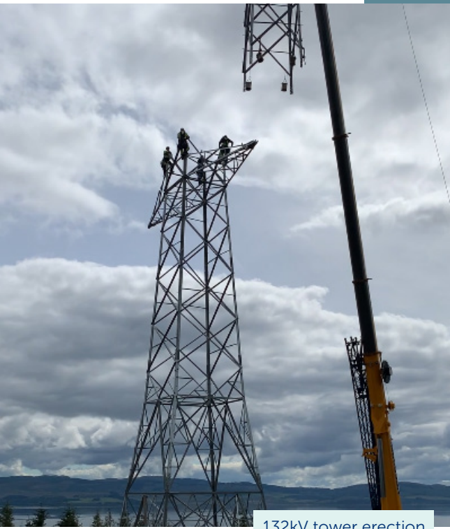
132kV tower erection
