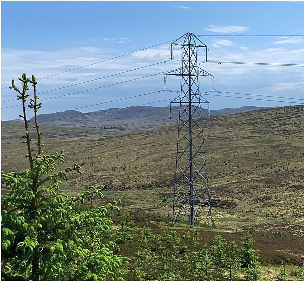
Photo 1.1: Steel lattice tower design
