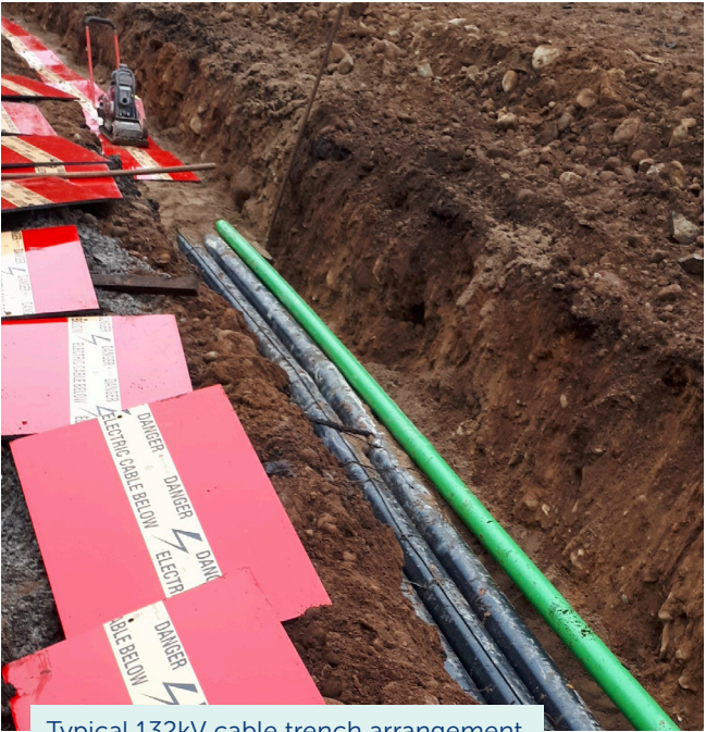
Typical 132kV cable trench arrangement
