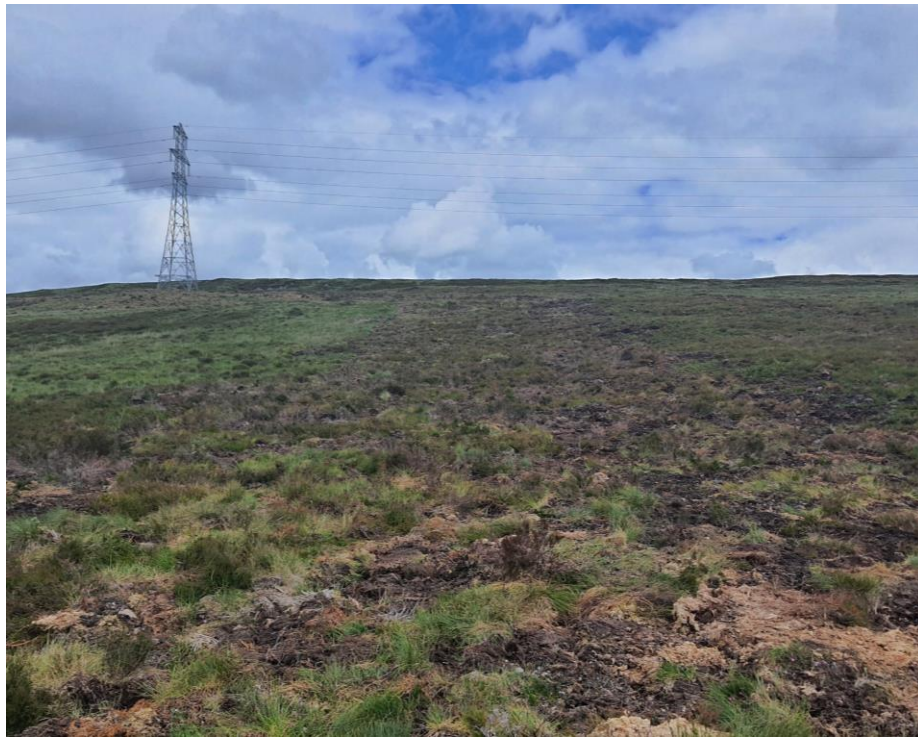
Photo 1: Reinstatement of temporary track using turves.
