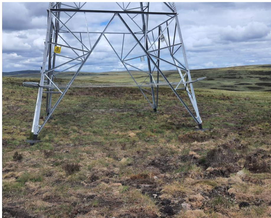
Photo 2: Example of reinstatement around tower foundations.
