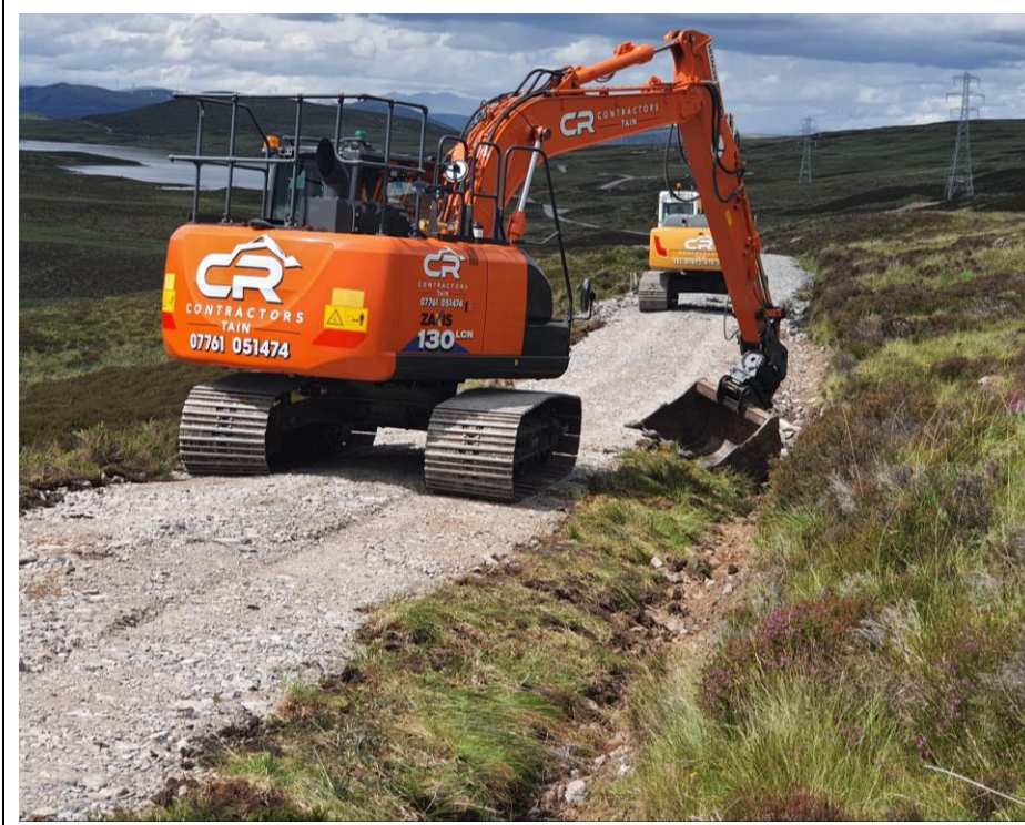
Photo 4: Formation of an access track verge using whole turns.
