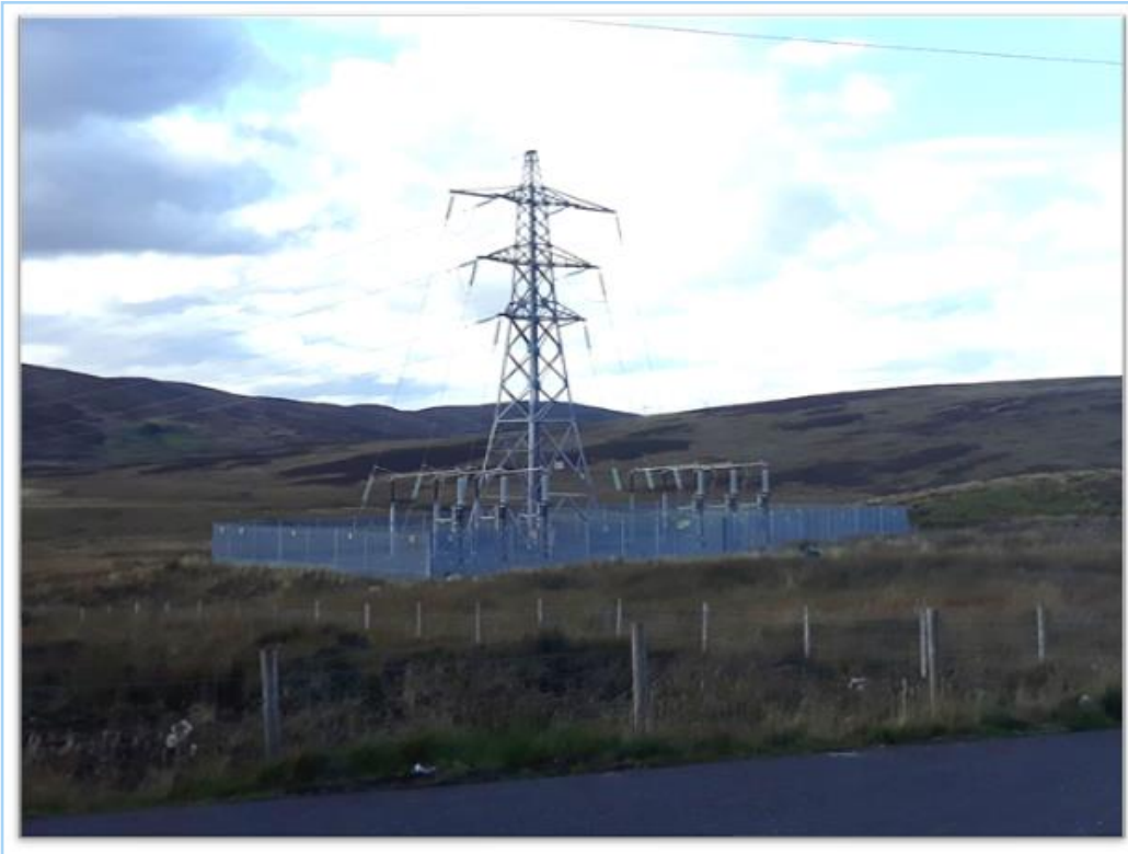
Plate 1.2: Example of a Cable Sealing End Compound
