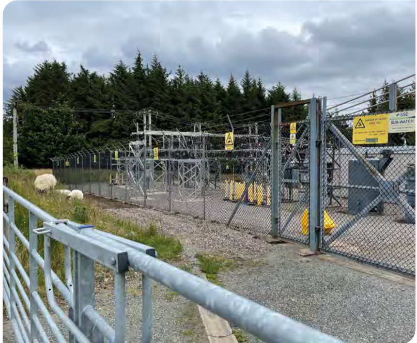
Existing Broadford Substation looking eastwards
