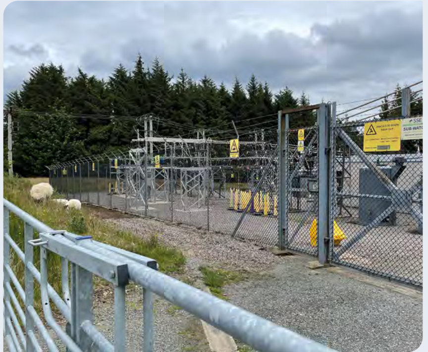
Existing Broadford Substation looking eastwards
