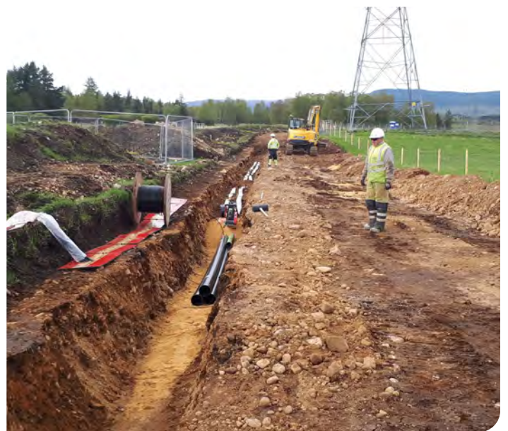
Figure 3 An Example of Underground Cable installation
