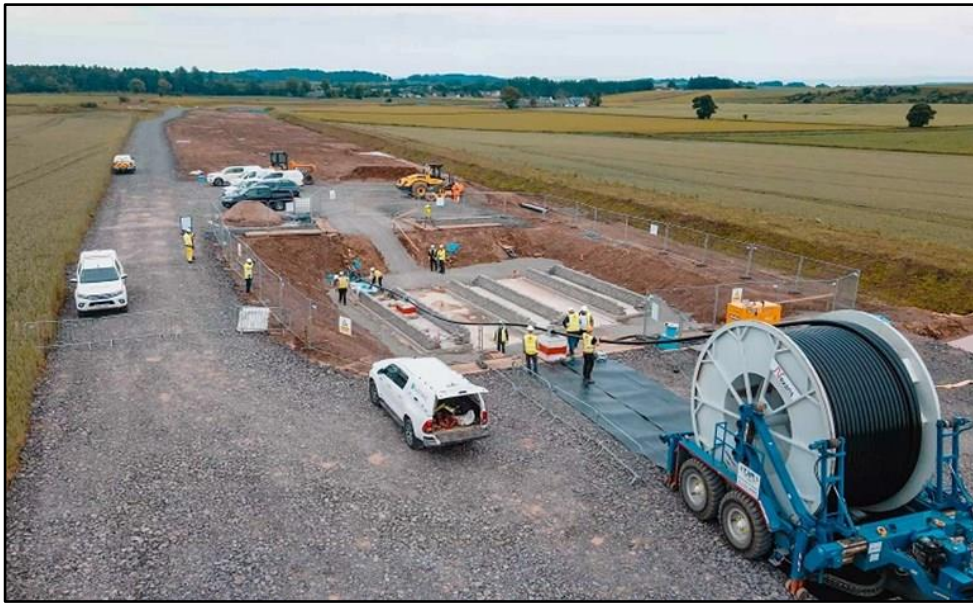
Plate 2.5: Photograph of Underground Cable Installation
