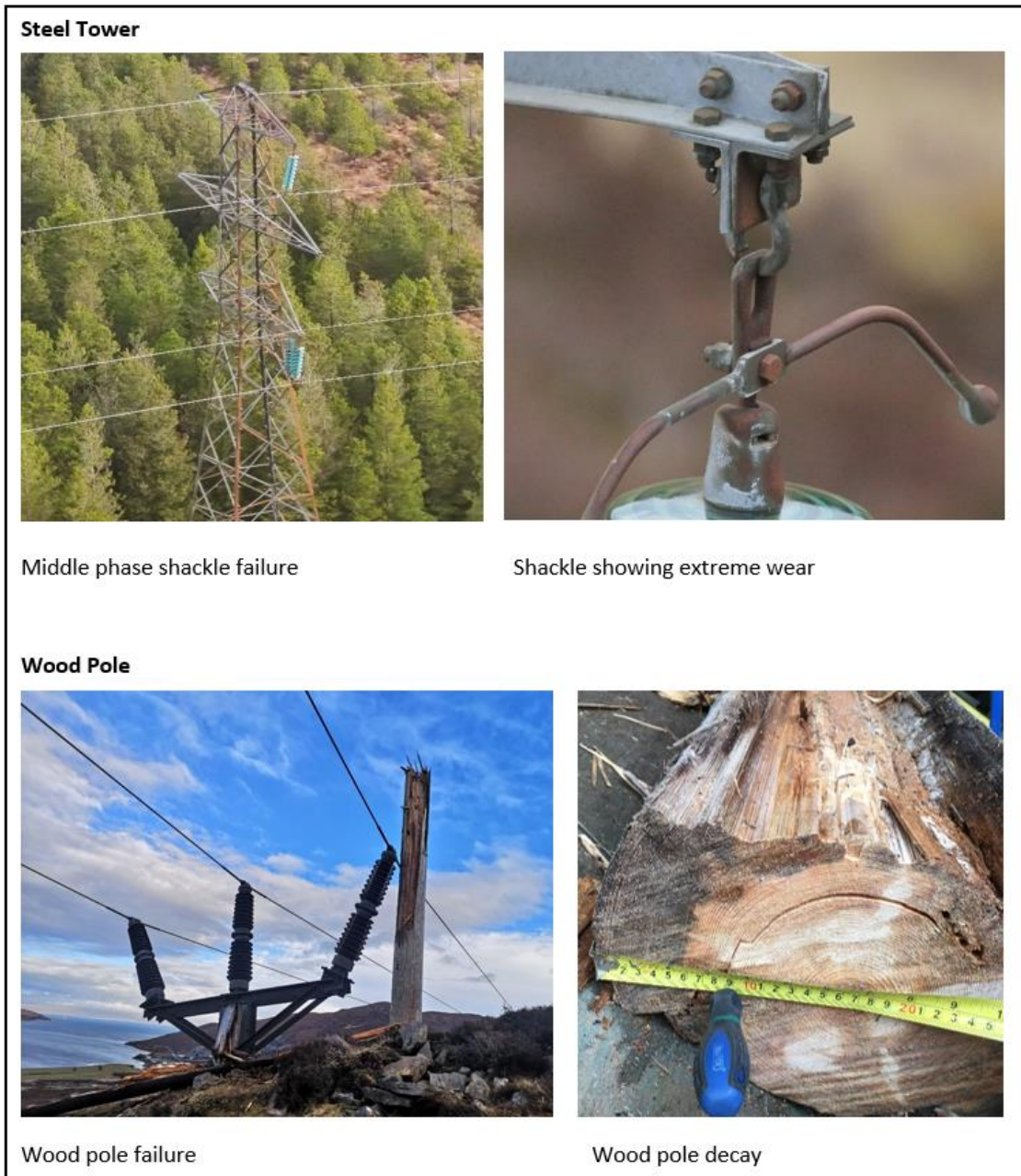
Plate 1.3: Photographs showing the condition of assets on the existing OHL
