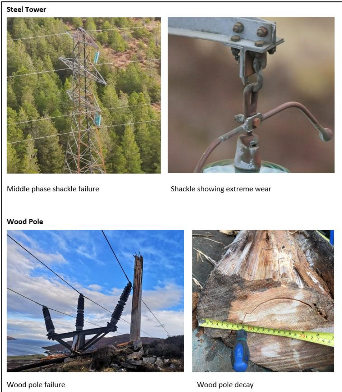
Plate 2.1: Photographs showing the condition of assets on the existing OHL
