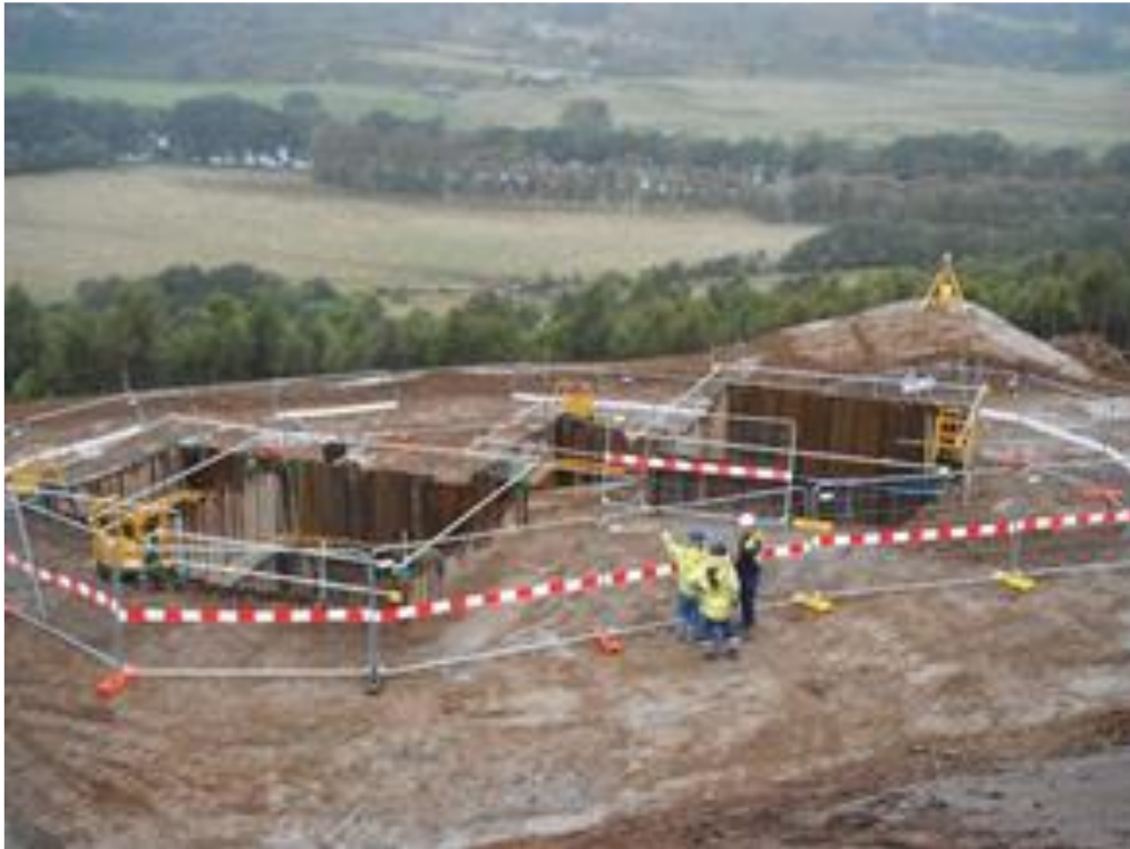
Tower Construction – Steel Lattice Towers
