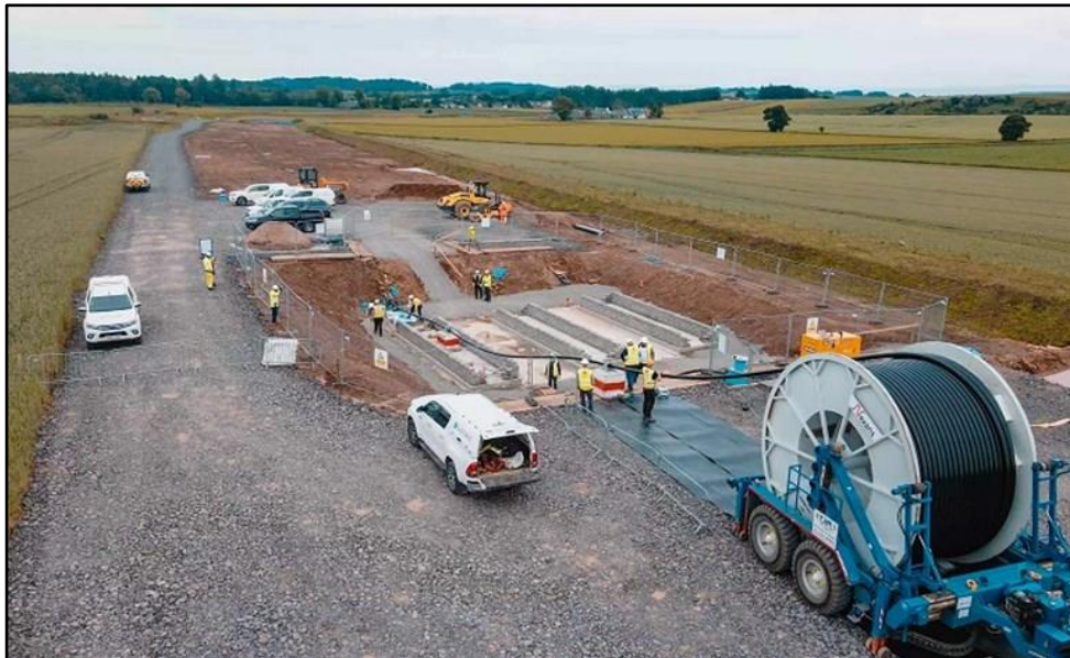
Plate 3.7: Photograph of Underground Cable Installation
