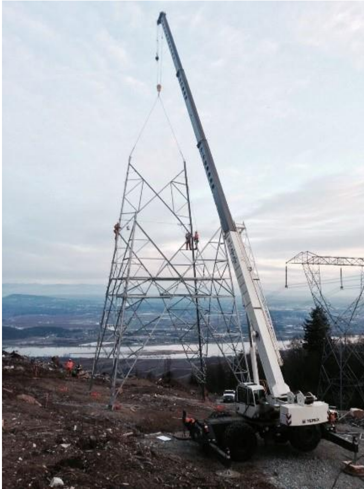
Plate 3.6: Illustrative Image of Steel Lattice Tower Construction
