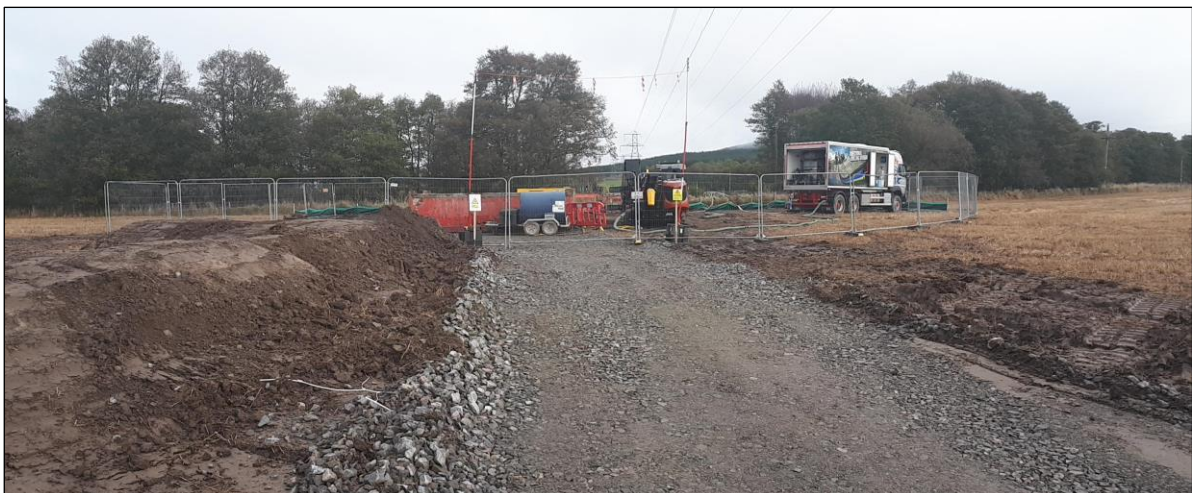
Plate 3.10: Example HDD Compound
