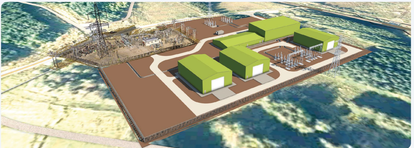
A 3D model drawing of the existing substation layout (left hand corner) with the proposed extension beneath.
