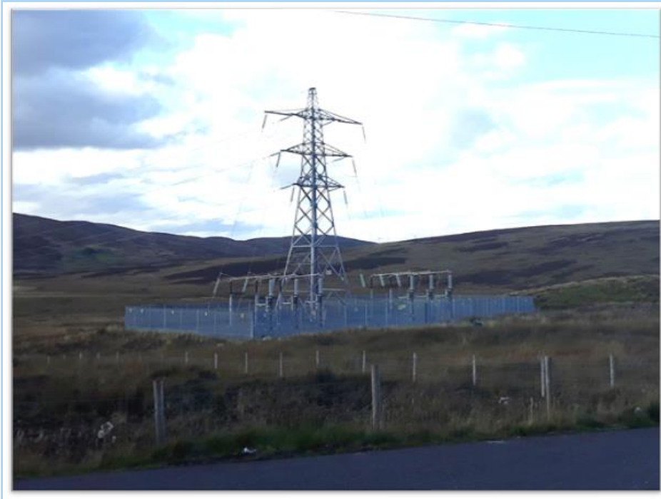
Plate 7.2: Example of a Cable Sealing End Compound
