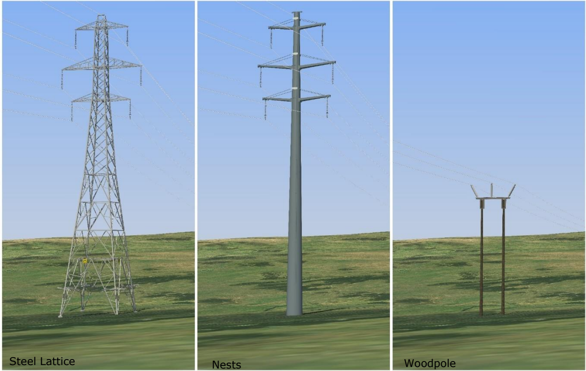
Plate 2.2: Example OHL Structures
