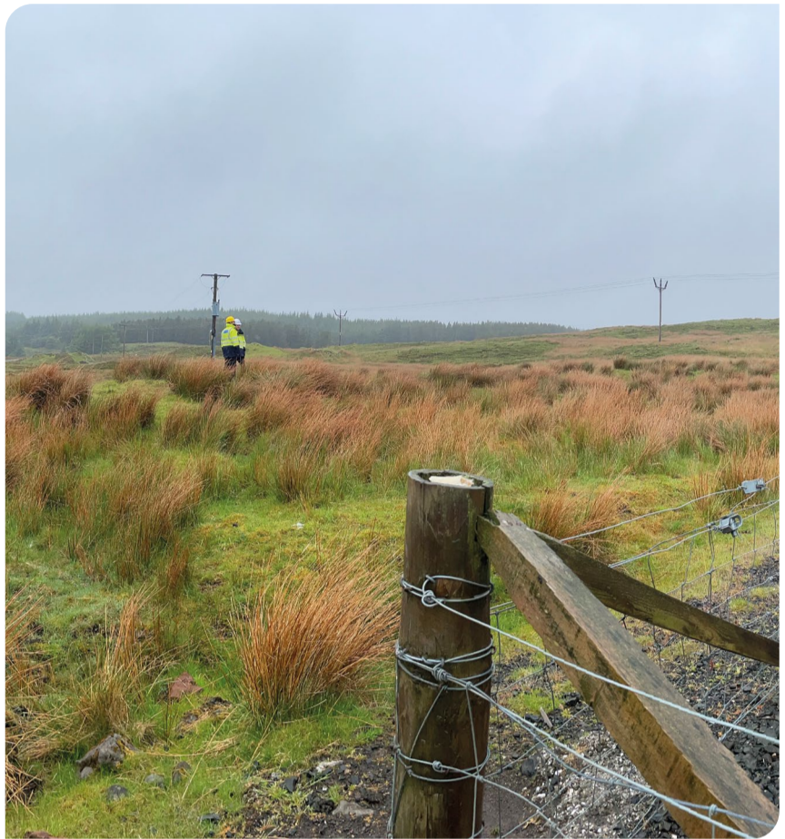
Eastern fenceline of the existing substation
