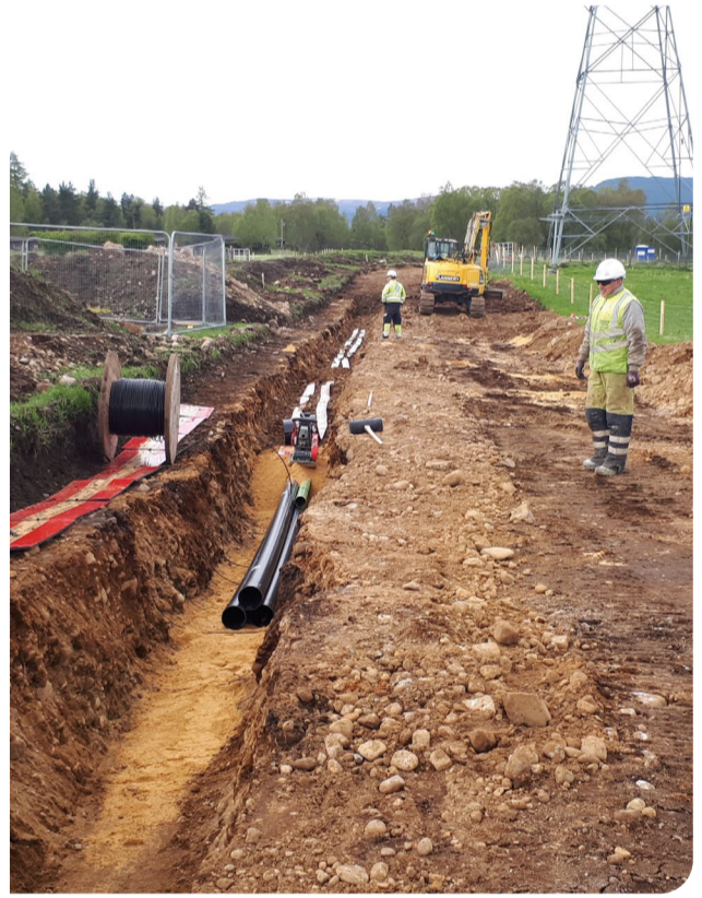
Figure 3 An Example of Underground Cable installation
