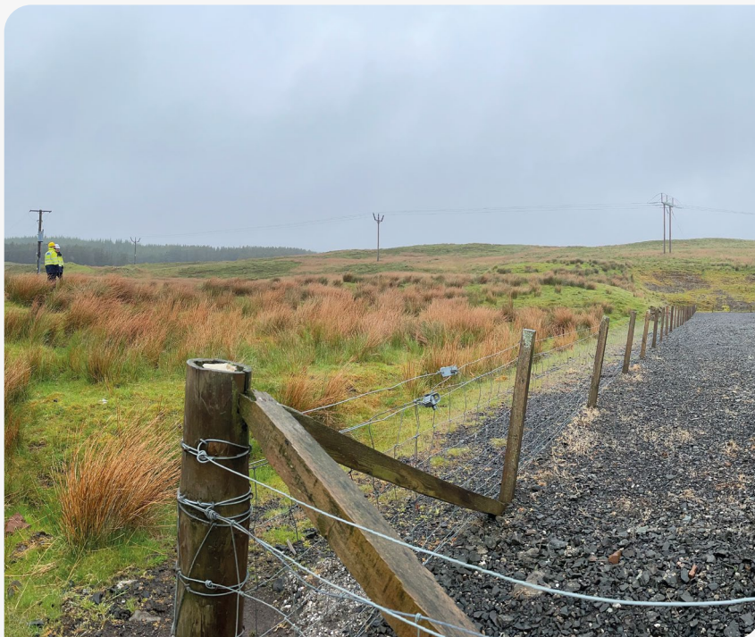
Eastern fenceline of the existing substation
