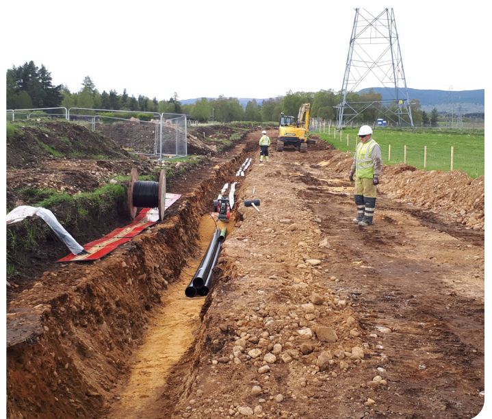
Figure 3 An Example of Underground Cable installation
