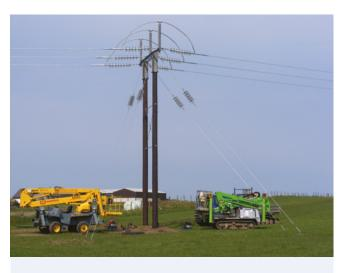
Above is a typical example of an angle wood pole which requires additional stays. Note that stays are not usually required on non-angle poles unless ground or weather conditions dictate.
