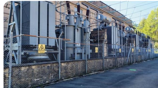
Engineering standards were very different when the transformers were installed in the 1990s. Modern transformers are quieter and more efficient but also require more space around them for cooling and for safe maintenance access.
