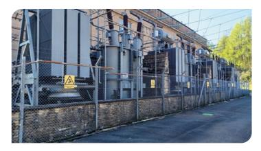
Engineering standards were very different when the transformers were installed in the 1990s. Modern transformers are quieter and more efficient but also require more space around them for cooling and for safe maintenance access.
