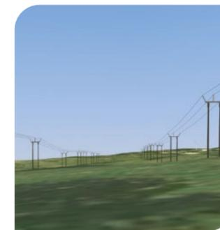
Two Single Circuit Trident Low Profile OHLs To be utilised for the connection between Kergord – Gremista / Mossy Hill. These would be positioned in parallel, approx. 30-50m apart.
