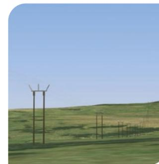
Single Circuit Trident Low Profile OHL. Standard Pole height is between 11-17m and pole spacings are in the range 70-100m.
