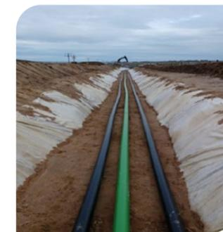
UGC power cables; either ducted or directly buried, in an underground trench nominally 1m below ground level.
