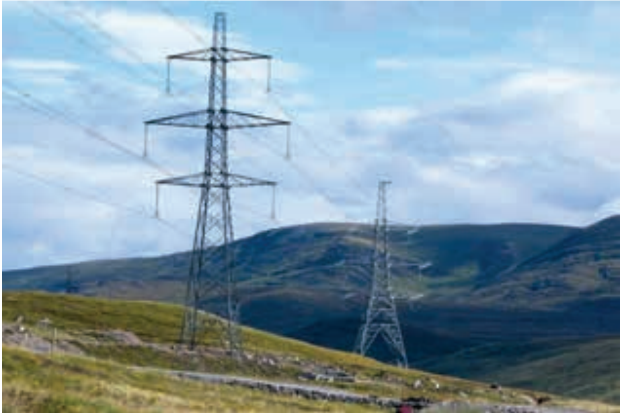
Plate 2.1 – Existing SSE400 steel lattice tower design
