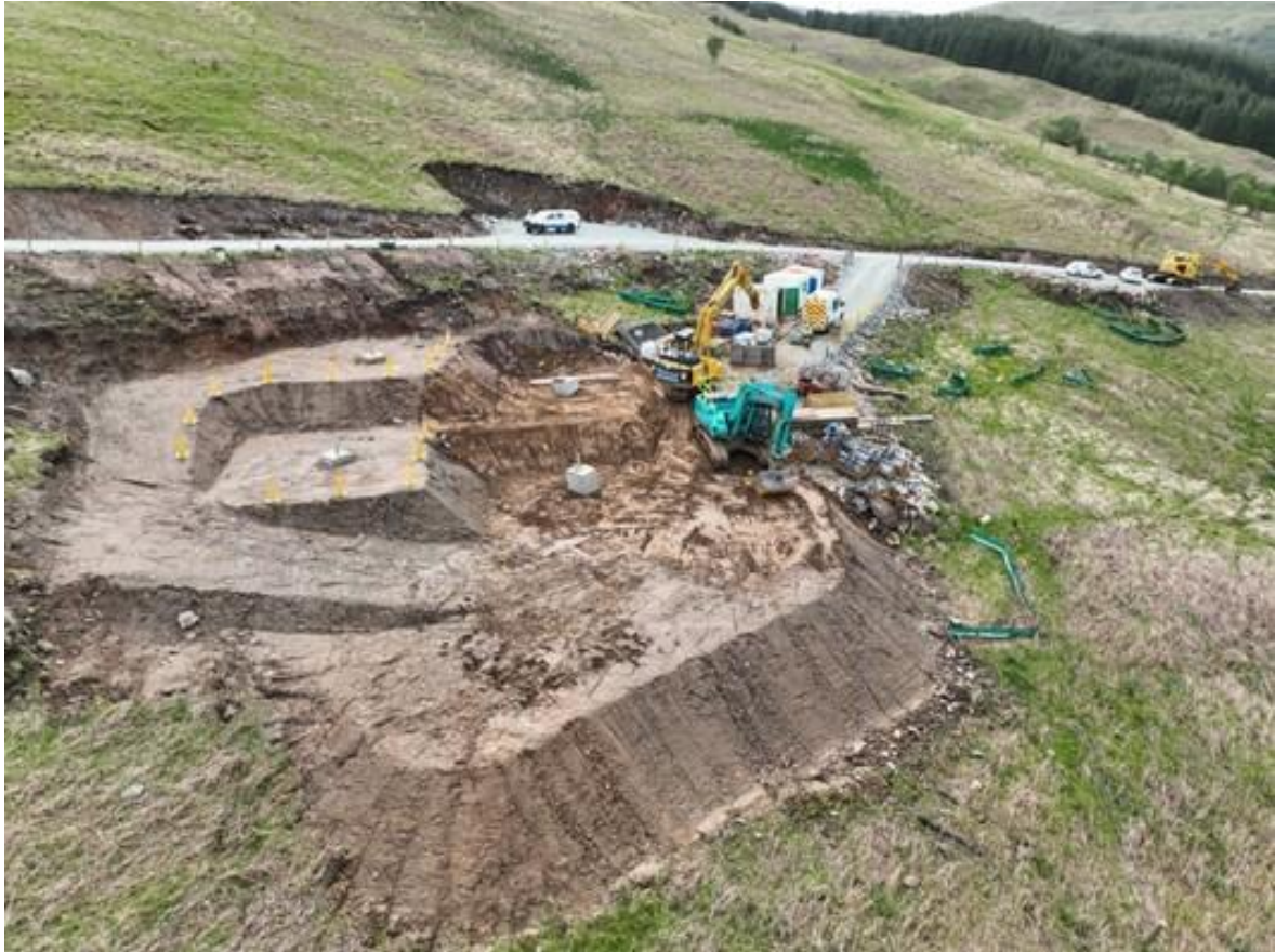
Plate 3.3: Illustrative Image of Tower Foundation Construction
