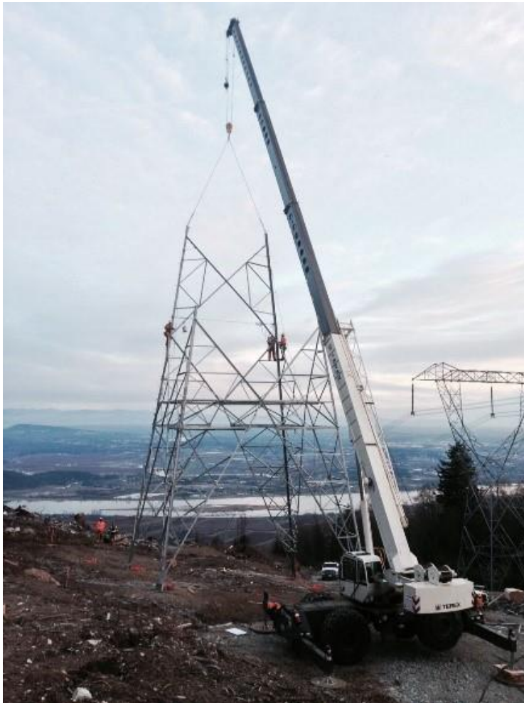
Plate 3.4: Illustrative Image of Steel Lattice Tower Construction
