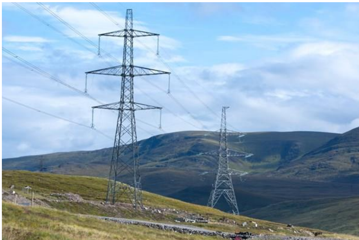
Plate 3.1: Existing AS4 Steel Lattice Tower Design
