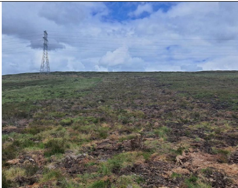
Photo 1: Reinstatement of temporary track using turves.
