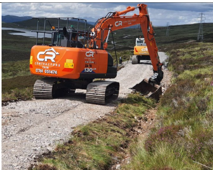
Photo 4: Formation of an access track verge using whole turves.
