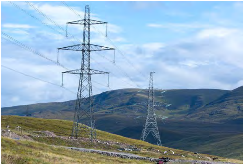
Figure 2.2 Existing AS4 Steel Lattice Tower Design
