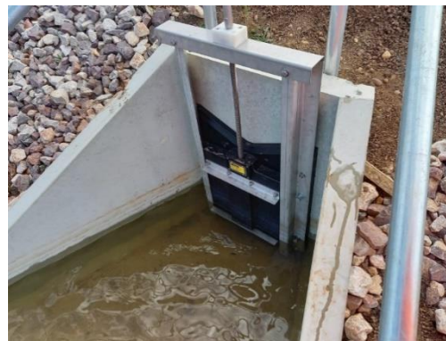
Figure 20: Example of final discharge penstock shutoff
