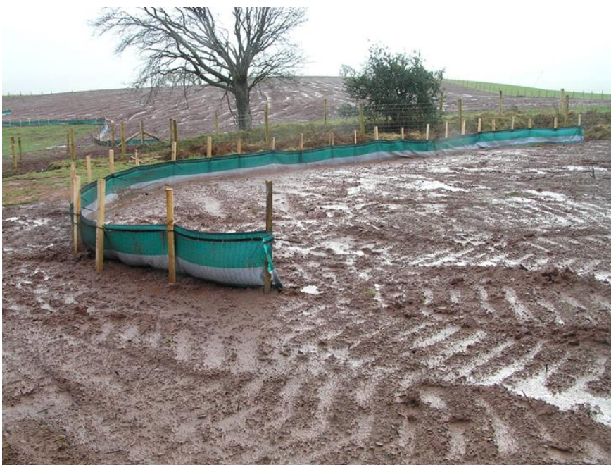
Figure 21: Example of silt fencing installation
