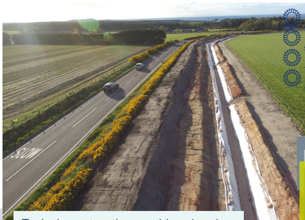
Typical construction corridor, showing haul road, trench and topsoil storage
