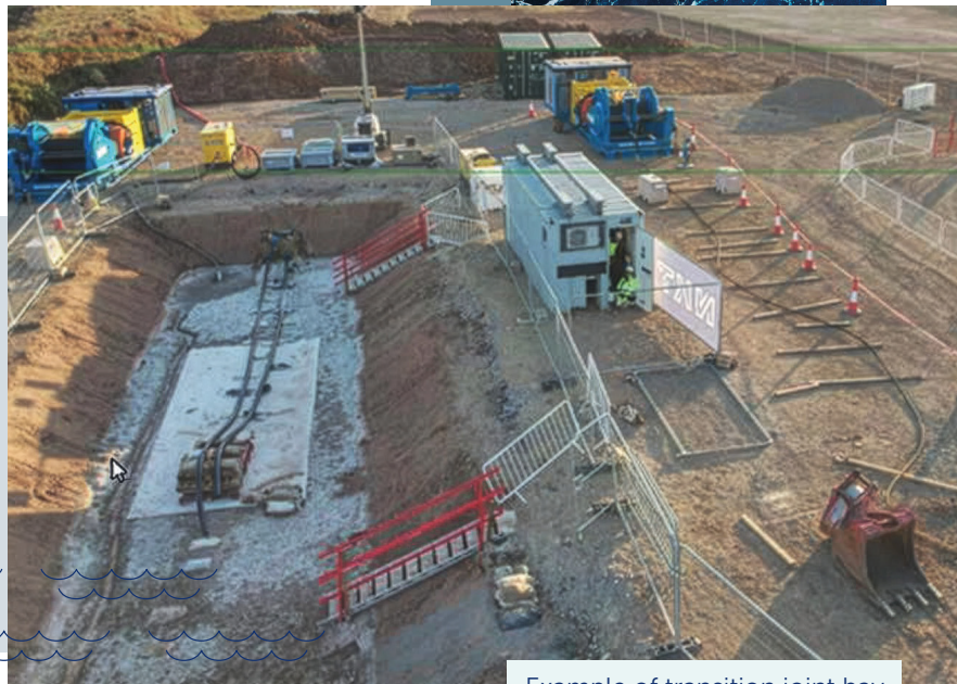
Example of transition joint bay
