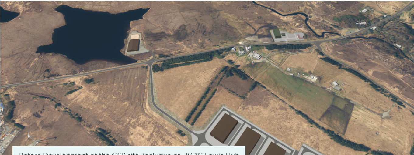
Before Development of the GSP site, inclusive of HVDC Lewis Hub
