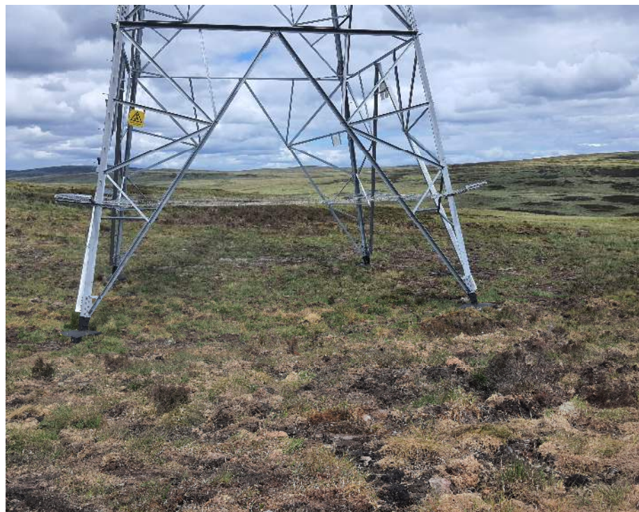
Photo 2: Example of reinstatement around tower foundations.
