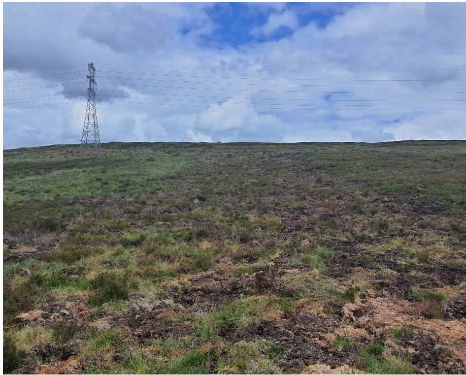
Photo 1: Reinstatement of temporary track using turves.
