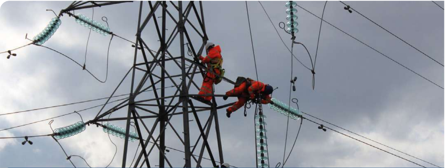
The above image shows the construction of a new steel lattice tower.
