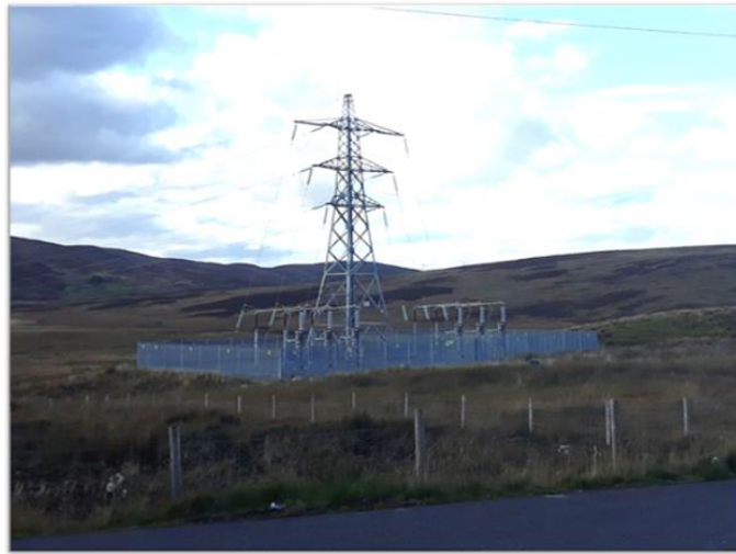
Plate 2.2: Typical Cable Sealing End Compound
