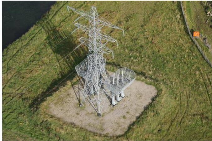
Plate 2.3: Typical Cable Sealing End Tower
