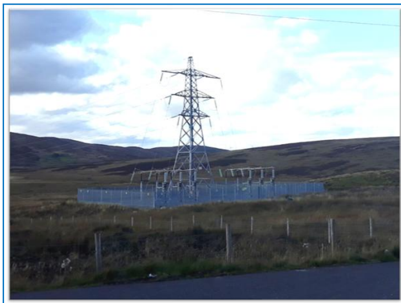
Plate 3.4: Example of a Cable Sealing End Compound
