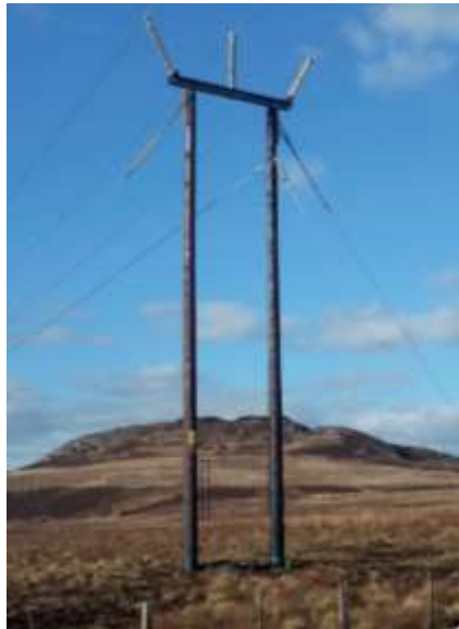
Plate 2.1 – Typical wooden trident pole design
