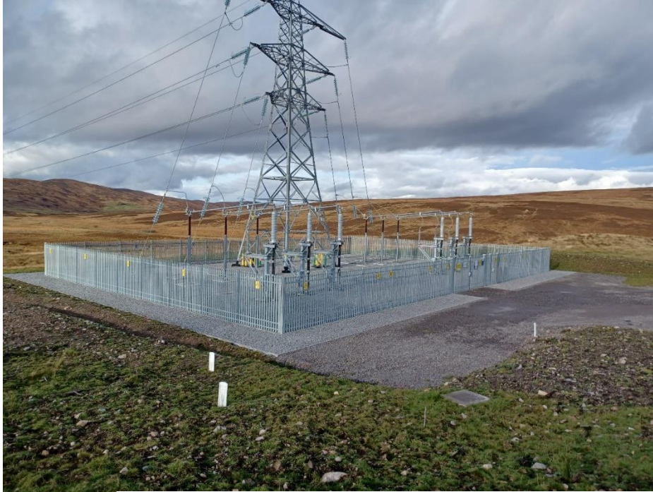
Plate 7.4 – Example of terminal tower with Sealing End Compound
