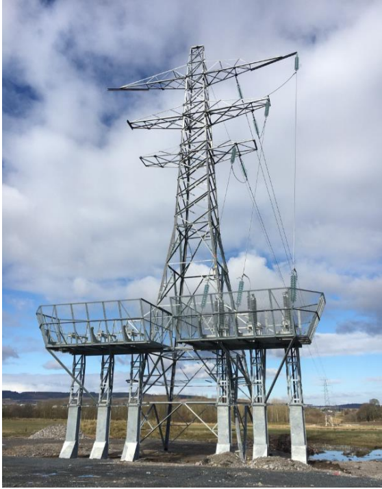
Plate 7.2 – Example of terminal tower with Sealing End Platform
