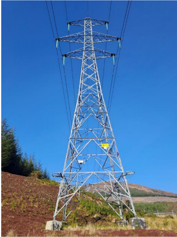
Plate 2.1 – Typical L7 steel lattice tower design
