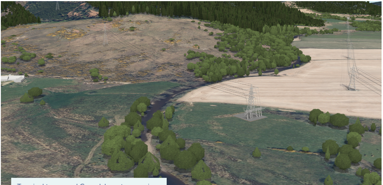
Terminal tower and Carradale water crossing
