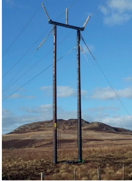
Plate 2.1 – Typical wooden trident pole design
