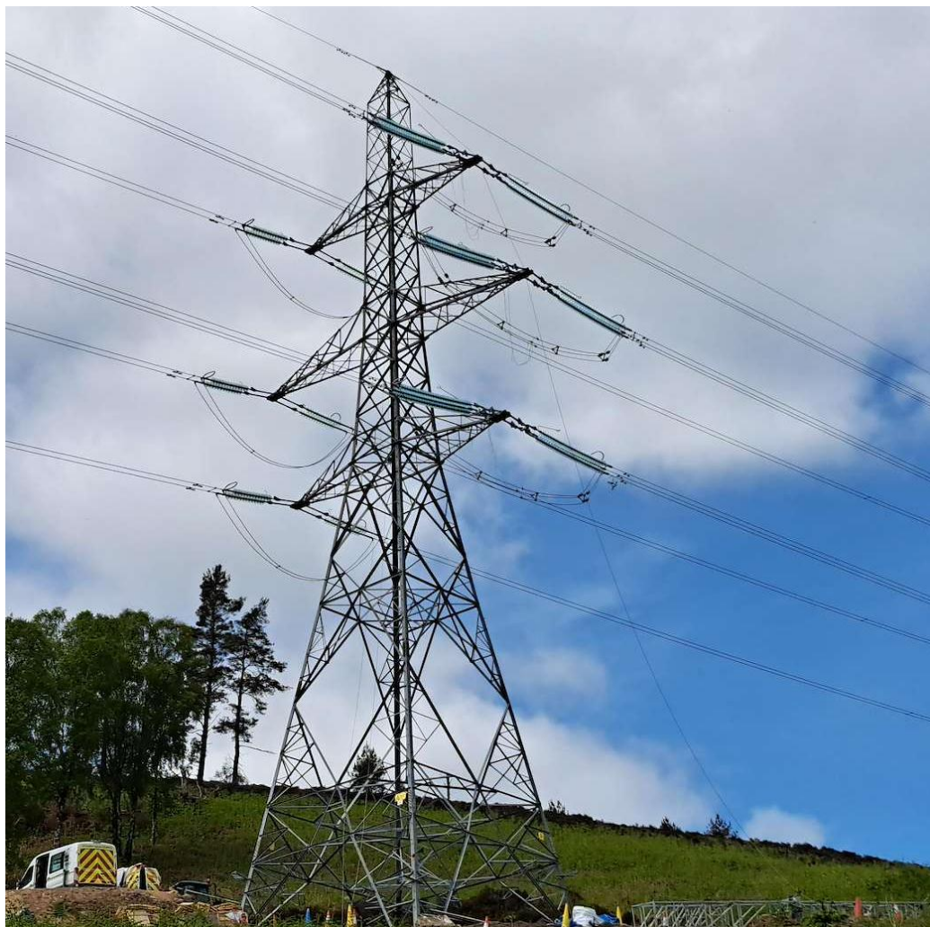
Plate 2-1: Typical steel lattice tower design (L8)
