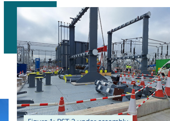
Figure 1: PST 2 under assembly
