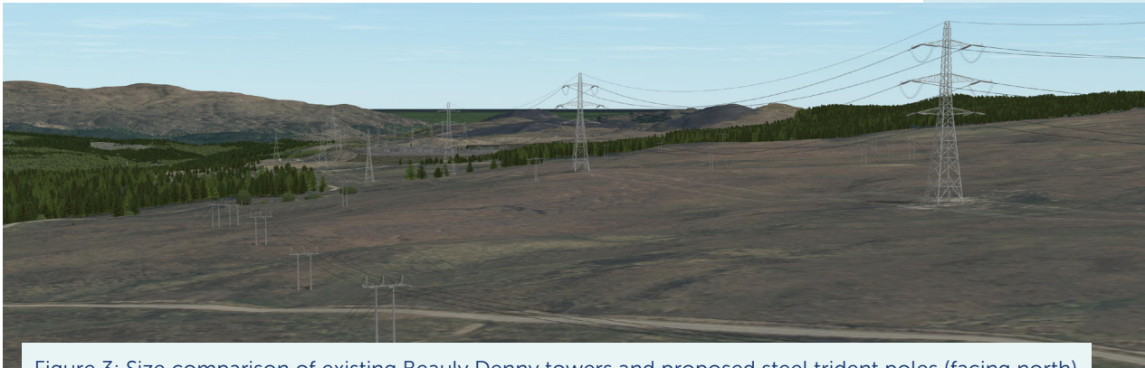
Figure 3: Size comparison of existing Beauly Denny towers and proposed steel trident poles (facing north)
