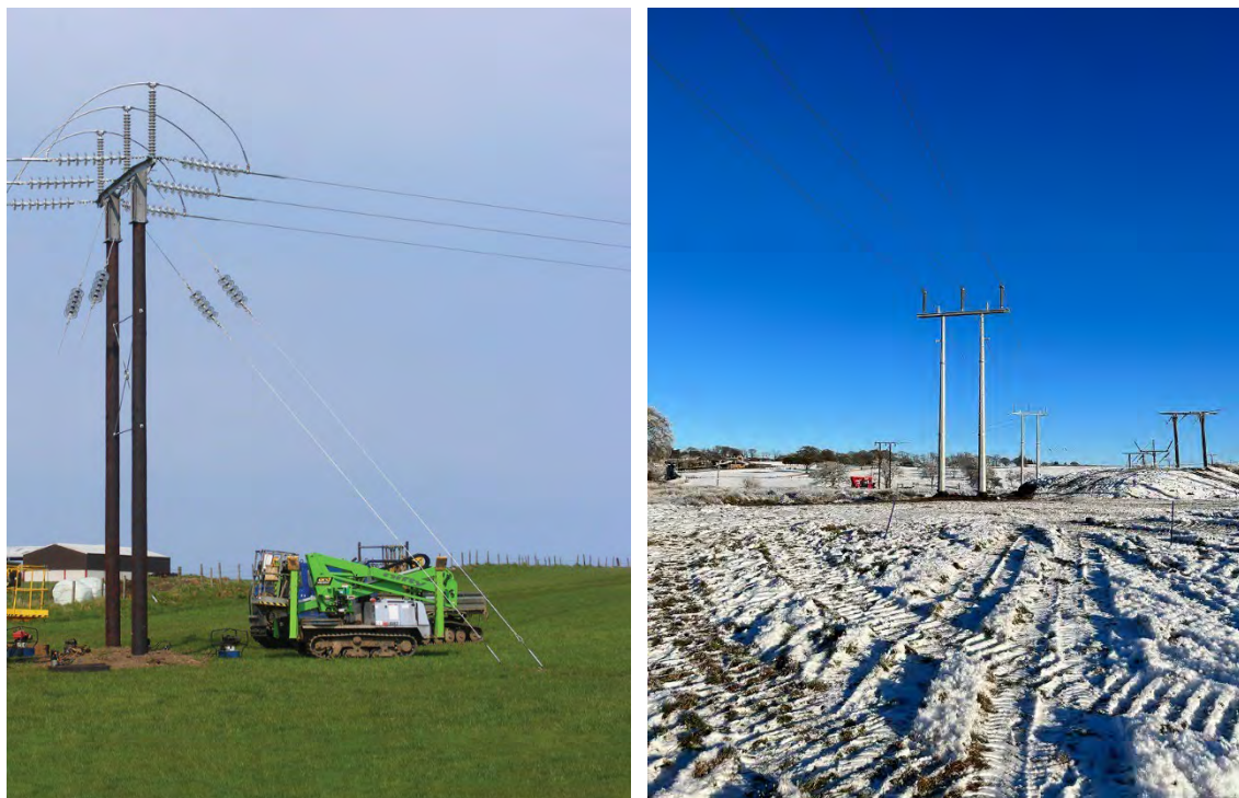
Figure 3-1 Typical layout of wood and steel trident poles
