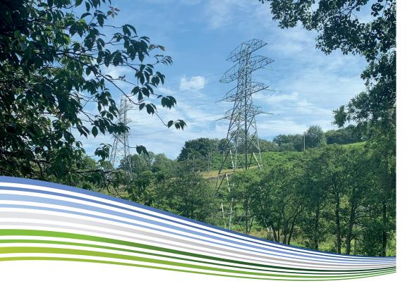
The overhead steel tower line which runs between Killin and Inveranan was constructed in 1952, with the section between Killin and St Fillans constructed in 1955, both sections are operated at 132,000 volts.
