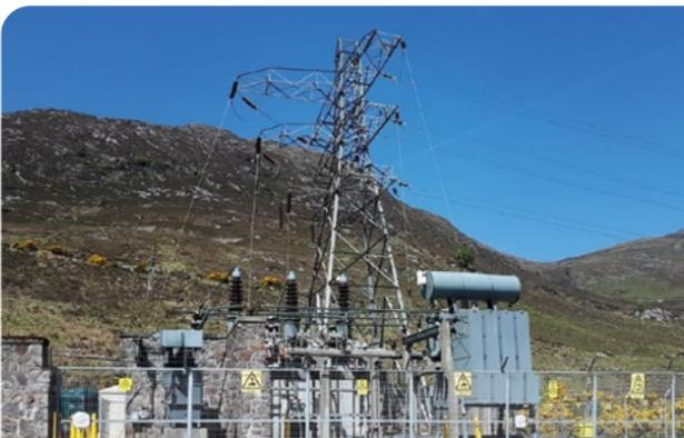
Existing external transformer arrangement needing to be replaced (at Deanie & Culligran)
