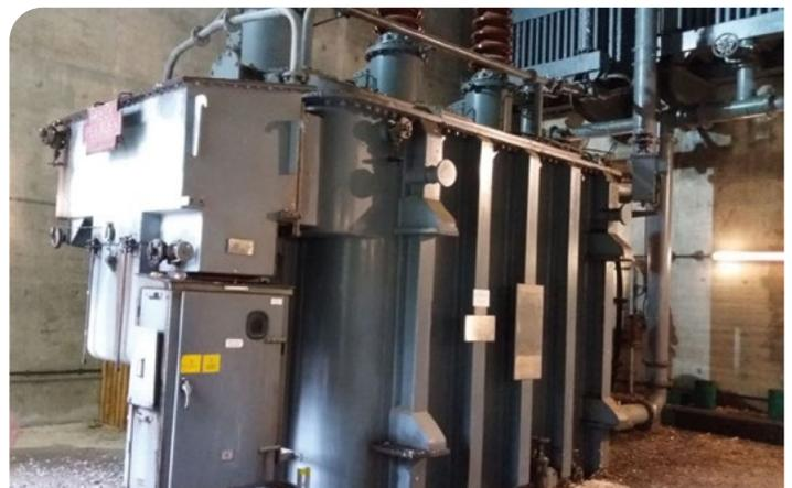
Existing internal transformers needing to be replaced (at Aigas & Kilmorack)
